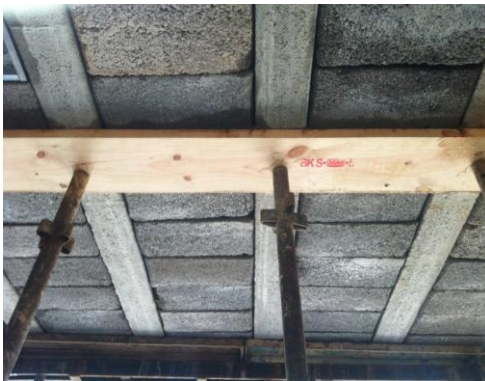
Typical/good rib & block propping
